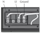
Connections for 230/240 VAC heater (4KW or 2 KW)
